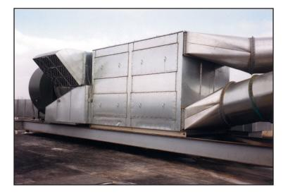
cant wheel for dehumidification. When the desiccant becomes saturated with moisture, they run hot air through it to regenerate the medium.
