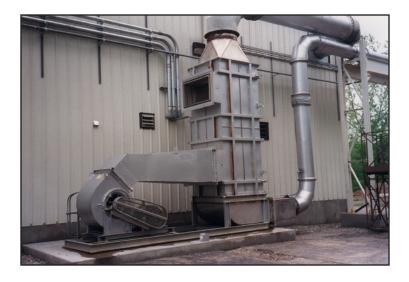
air comes from the process at  $900^{\circ}$ F – hot enough to burn the bags – and it must be cooled to  $250^{\circ}$ F. Previously, with the existing line, outside air was mixed with the hot air to cool it. A second line doing this would have resulted in exceeding the baghouse capacity.
