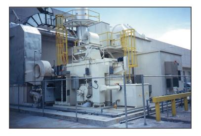
turned to Plymouth, Michigan-based Durr Environmental, a manufacturer of air pollution control systems that had previously supplied equipment for the facility. Des Champs supplied the VariMax<sup>™</sup> system, an indirect-fired recirculating gas heater. A burner in the combustion chamber generates heat, and the combustion products recirculate by means of a fan, rather than flowing straight up a stack.
